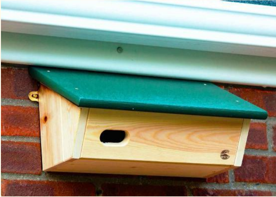
Figure 3. New swift box on side of village hall.
